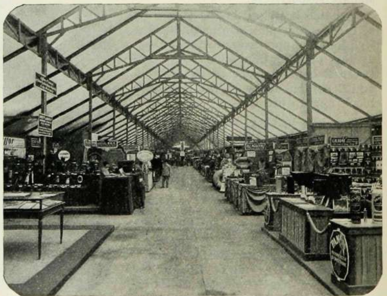
R 1330 View of the International Fire Protection Exhibition in Paris 1929. The Ericsson section is to the left.
