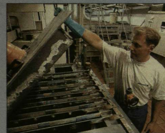
More environmentally friendly plant A new treatment plant was built when the plant was expanded. Lasse Hansson shows how copper residues from the process water are extracted so that the remaining water can be recirculated in the closed system. The extracted copper is sold and reused.
