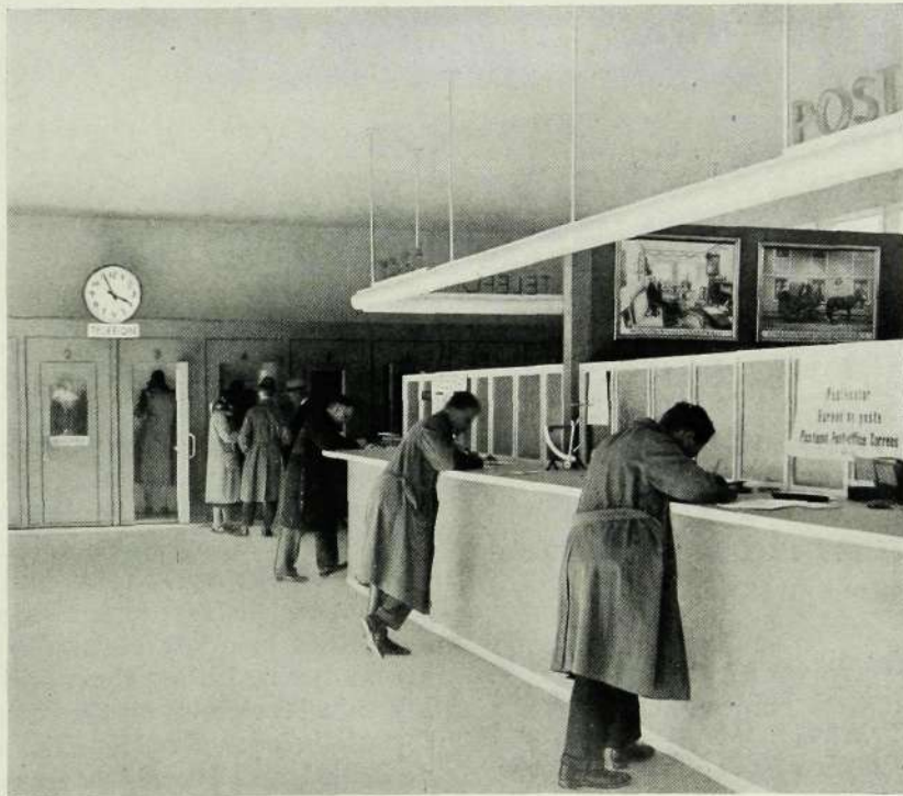
Interior view of the Public Rooms Building.
