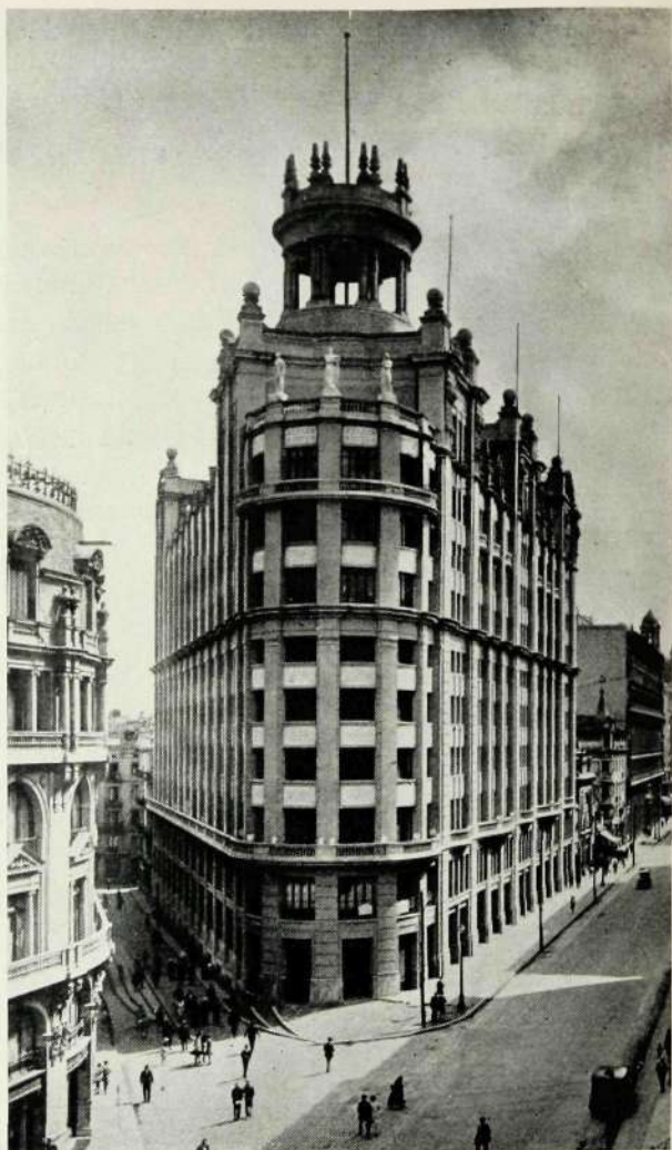
R 1695 View of the building, Layetana 18, Barcelona.
