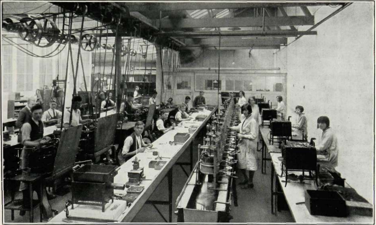
Ericsson Telephone Works—Switchboard Plug Moulding and Finishing Department
