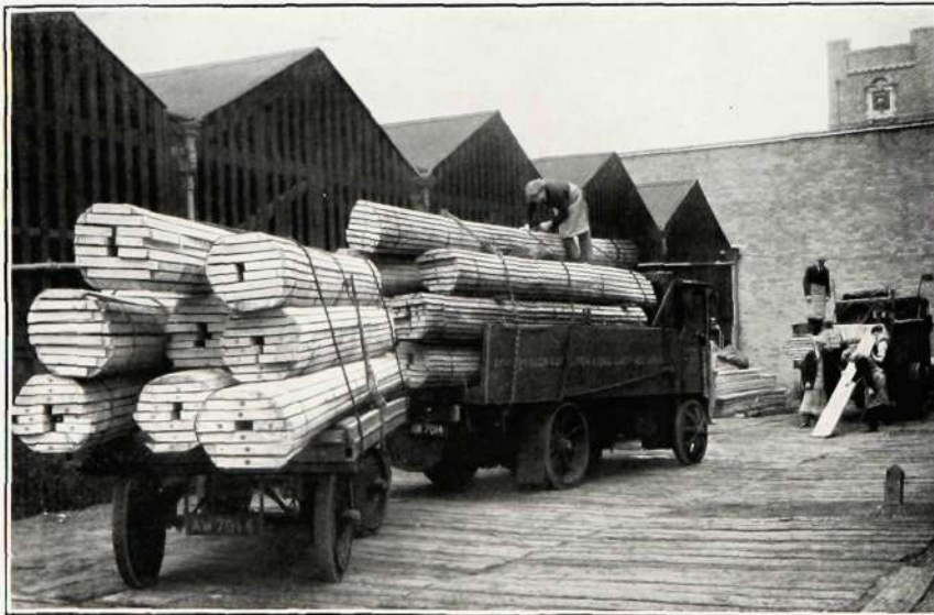
Timber Arriving at the Works
