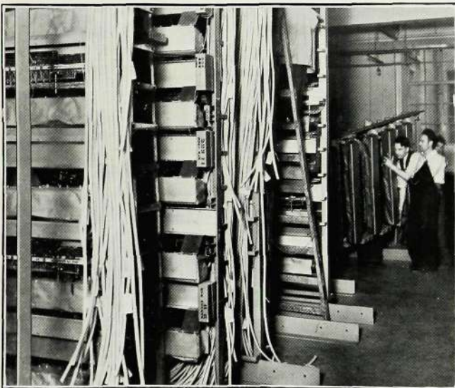
Fig. 5—Erecting Racks and Cables Run-in
