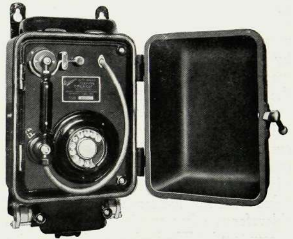
Fig. 1—Auto Mining Telephone with door open
