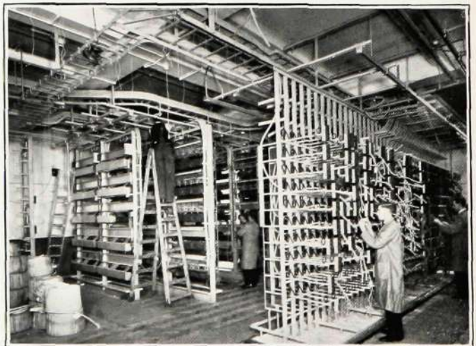
Fig. 4—Running Cables and Wiring Local Side I.D.F.
