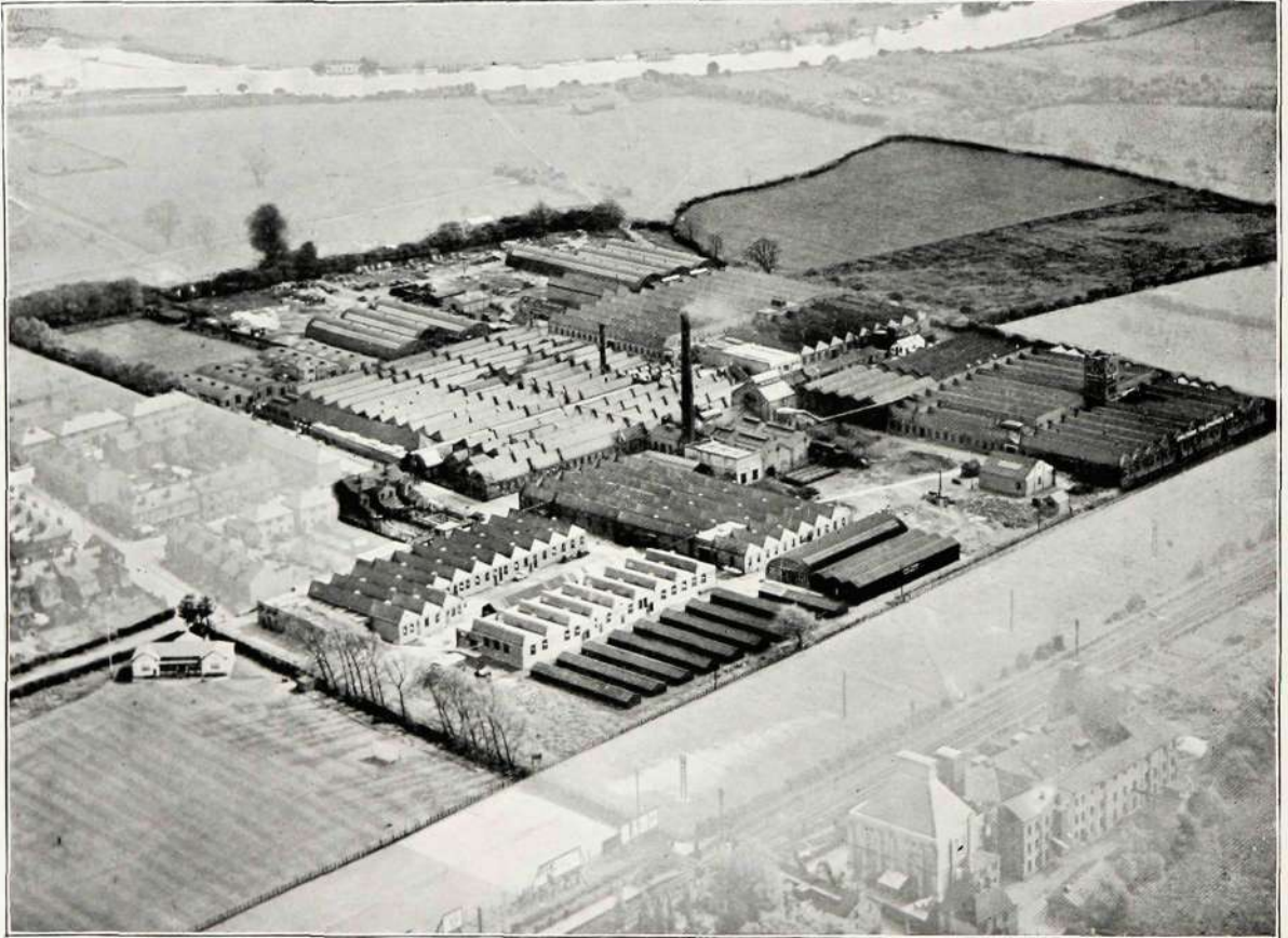
Aerial View of The Ericsson Works, Beeston, Nottingham
