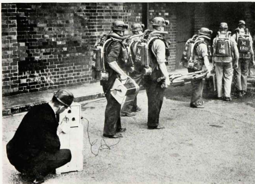
Fig. 3—Advance Party about to Commence Operations
