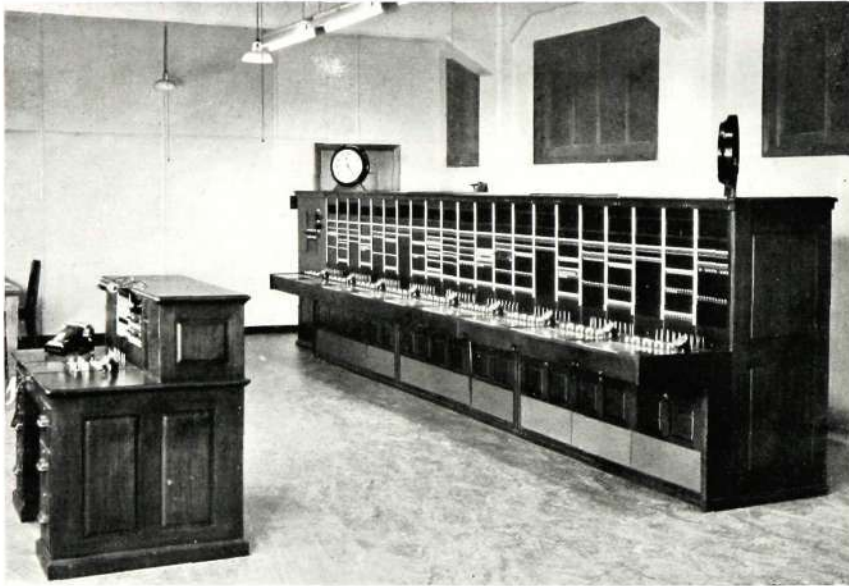
Fig. 2—Toll Switchboard and Supervisor's Desk.
