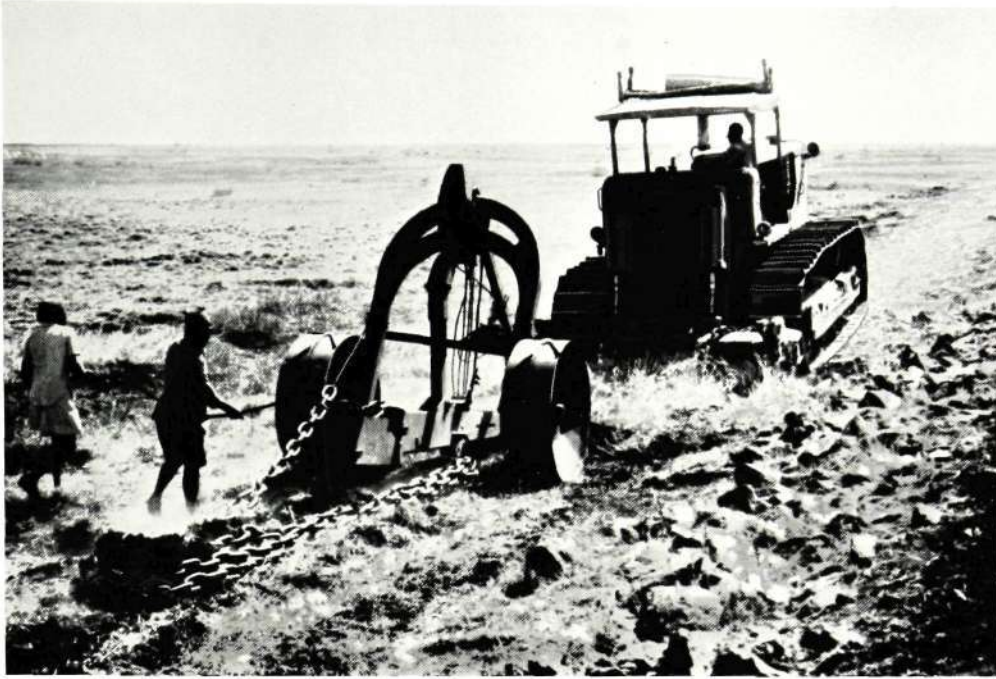
Figure 4—Cable-laying operations with tractor and plough
