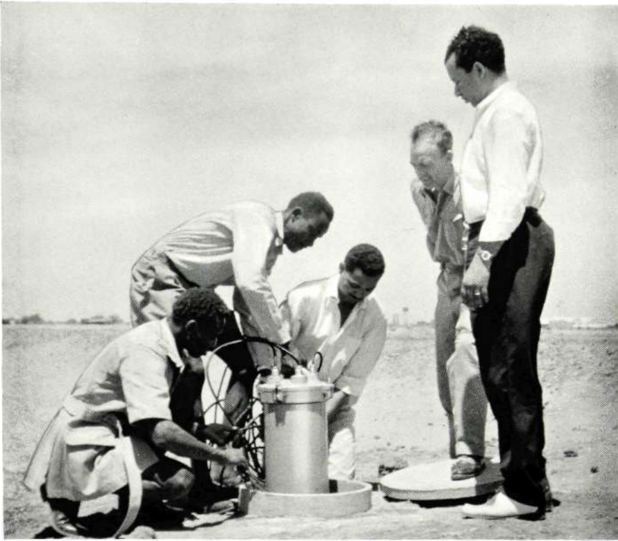
Figure 8—Engineers installing intermediate repeater (author 2nd from right)
