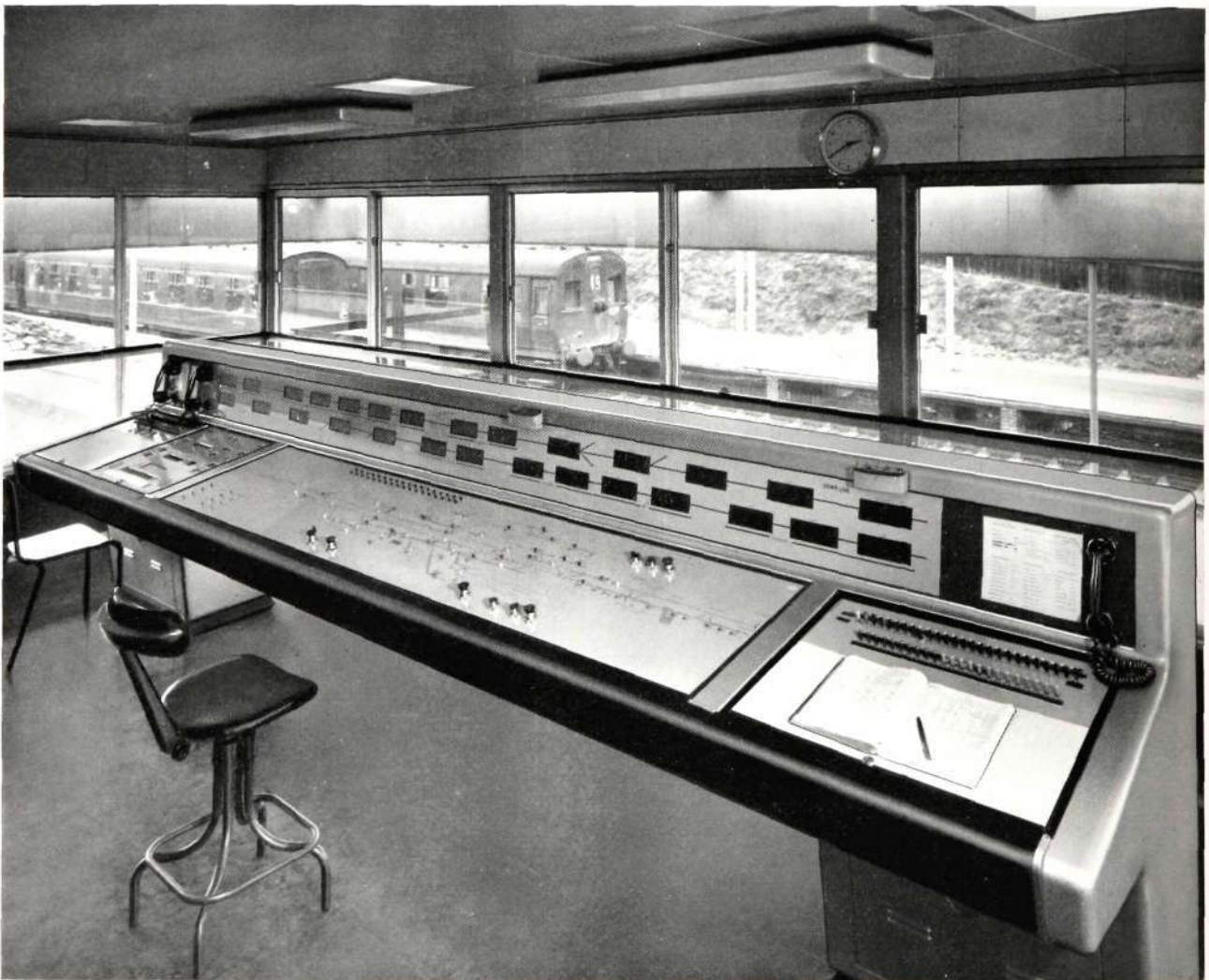
Figure 3—Power signalling control console
