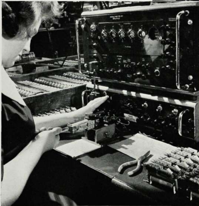
600-type relay coils in production on Aumann machines. One operator is here seen tending three winds. Plastic hats over the stationary spools 'funnel' the wire out from the spools to jockey wheels, thence to the machines.
