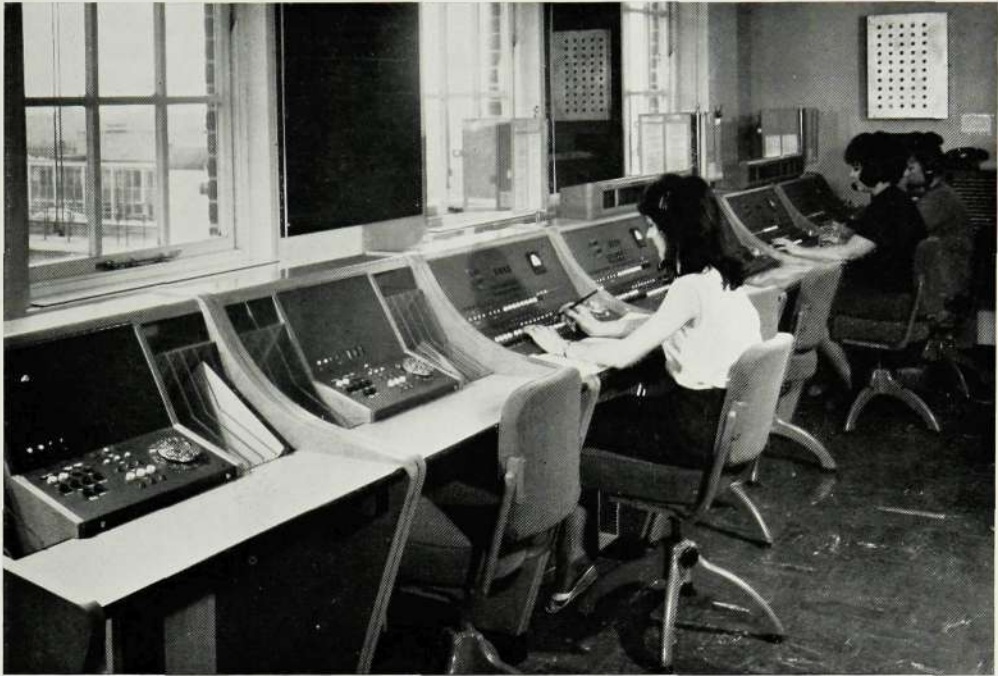
Figure 4—Part of the manual suite with two of the Room Service positions on the left
