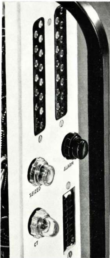
Figure 20—Front Panel of Incoming Supervisory Relay Set, showing (from top to bottom) monitoring sockets, signal lamps, call-trace neon lamp, and test jack
