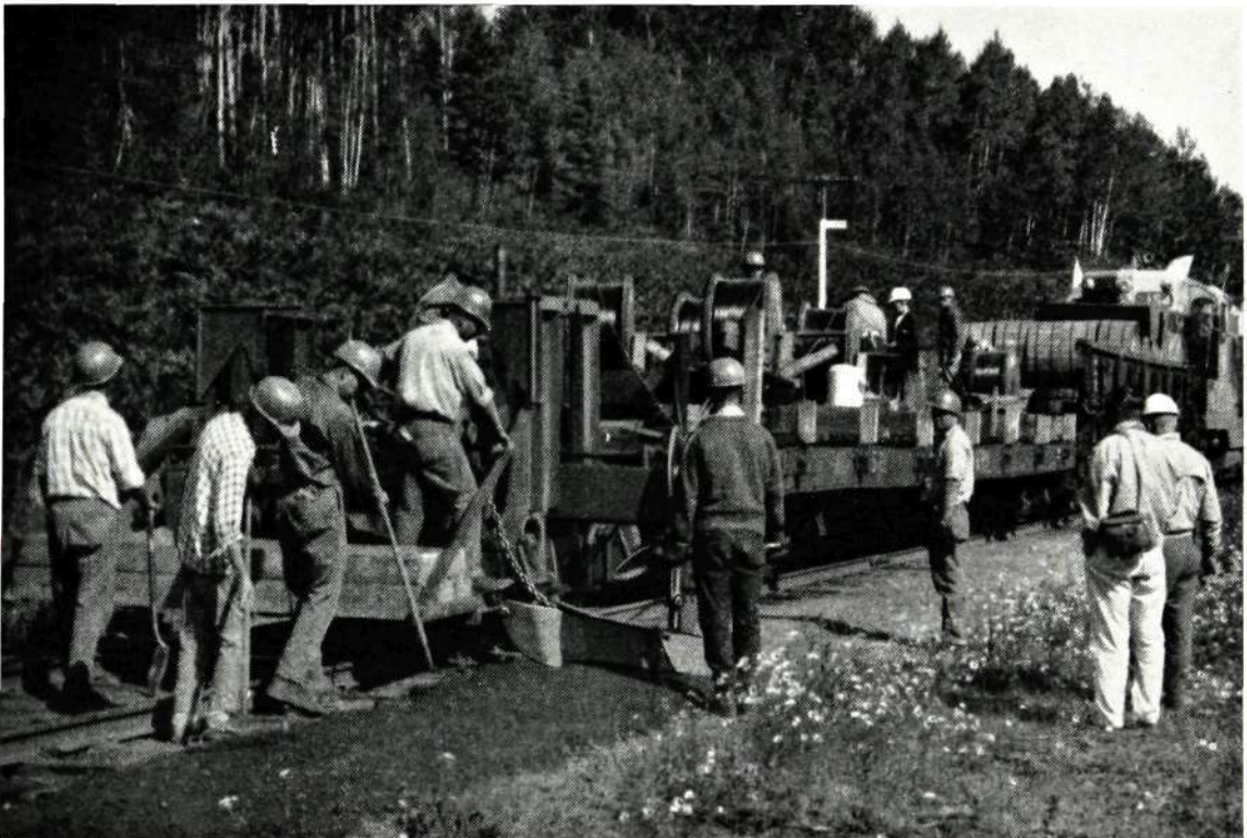
Figure 2—Cable-laying train with plough wagon at rear
