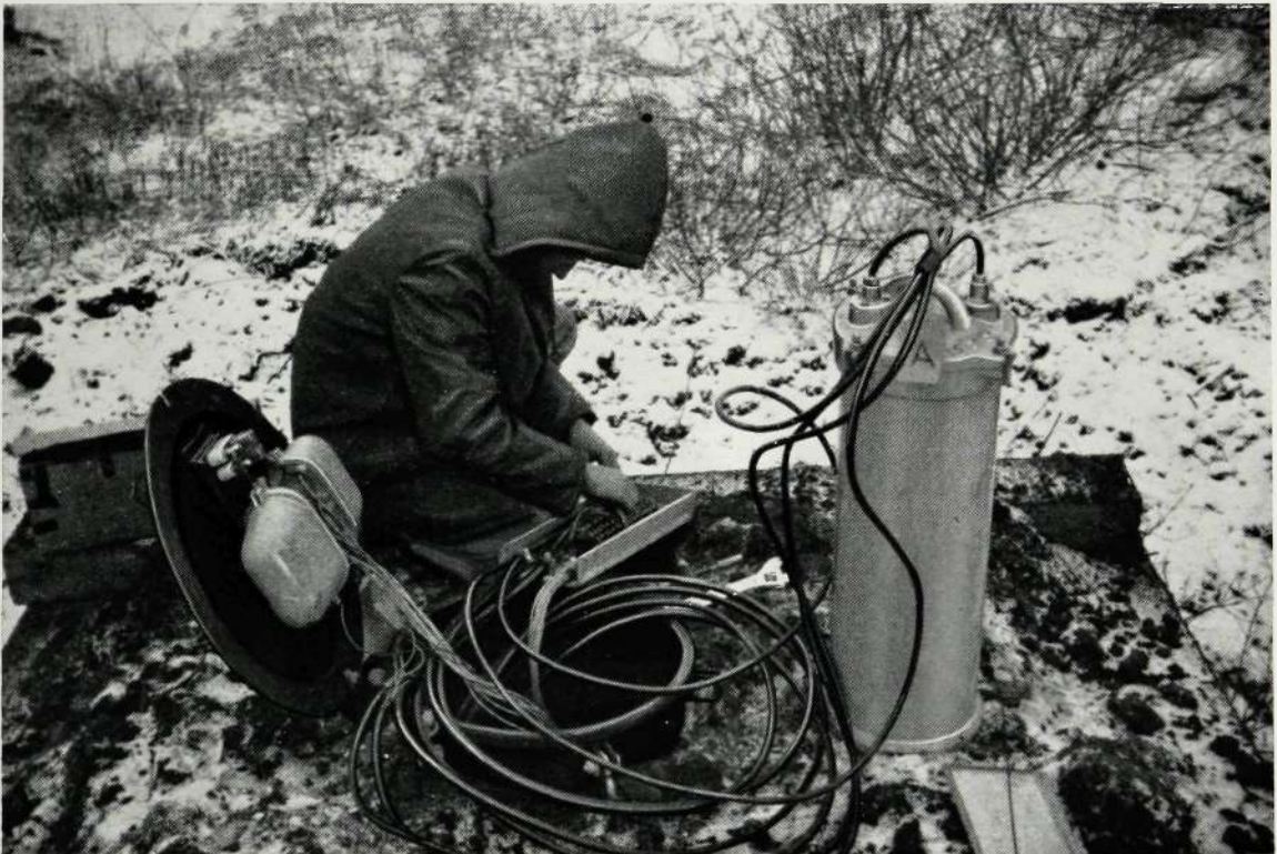
Figure 5—Terminating connections on open tag strip during installation of buried repeater
