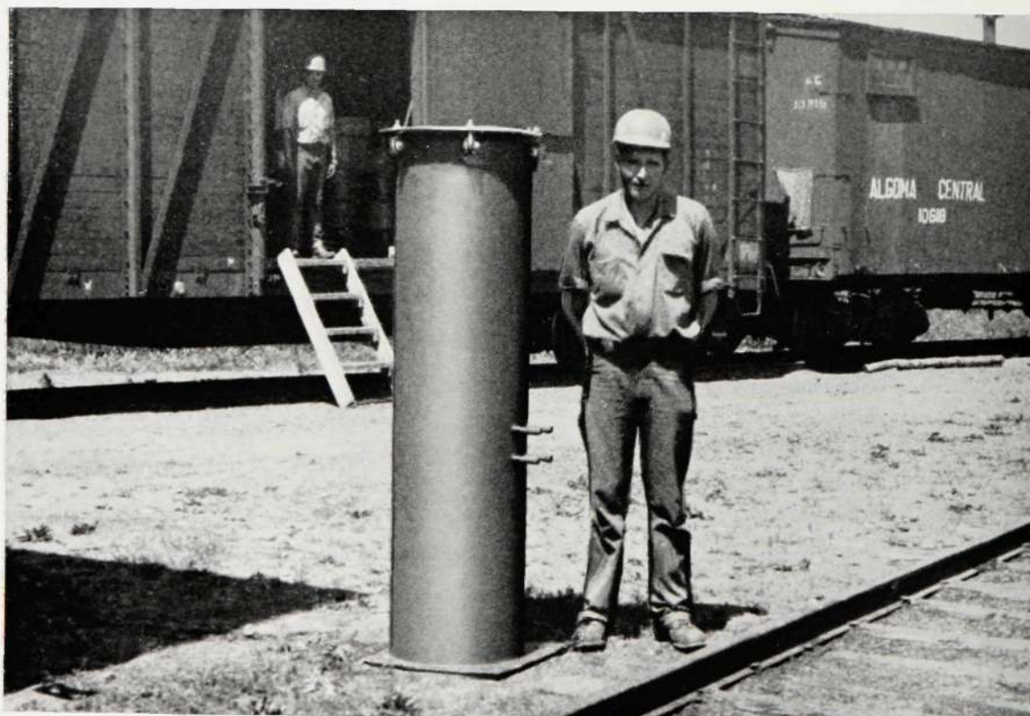
Figure 4—Manhole canister for installation on cable route
