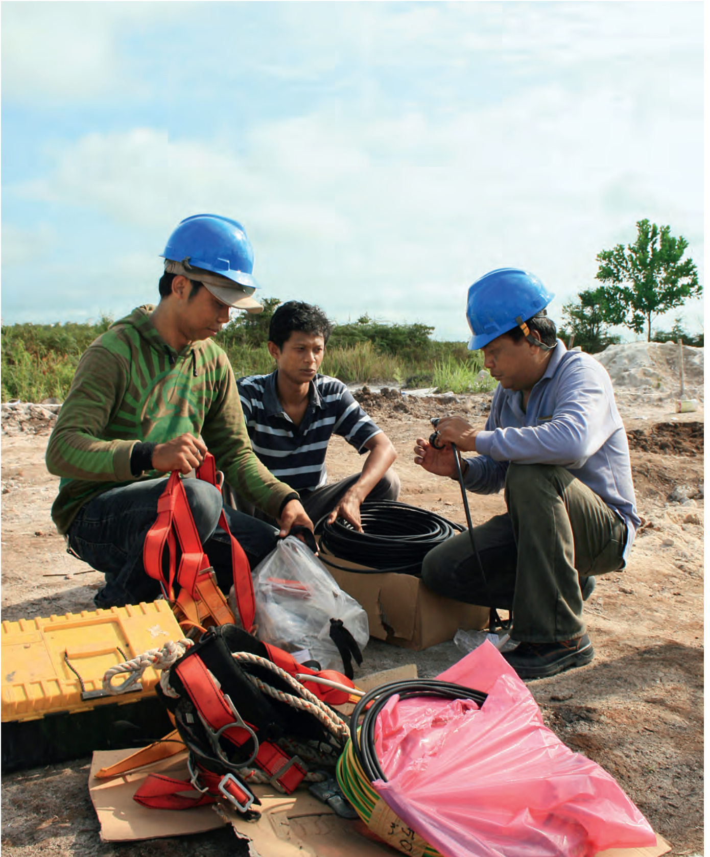
Kalimantan (Borneo), Indonesia. Ericsson's base station is coming together in the 34c heat.
