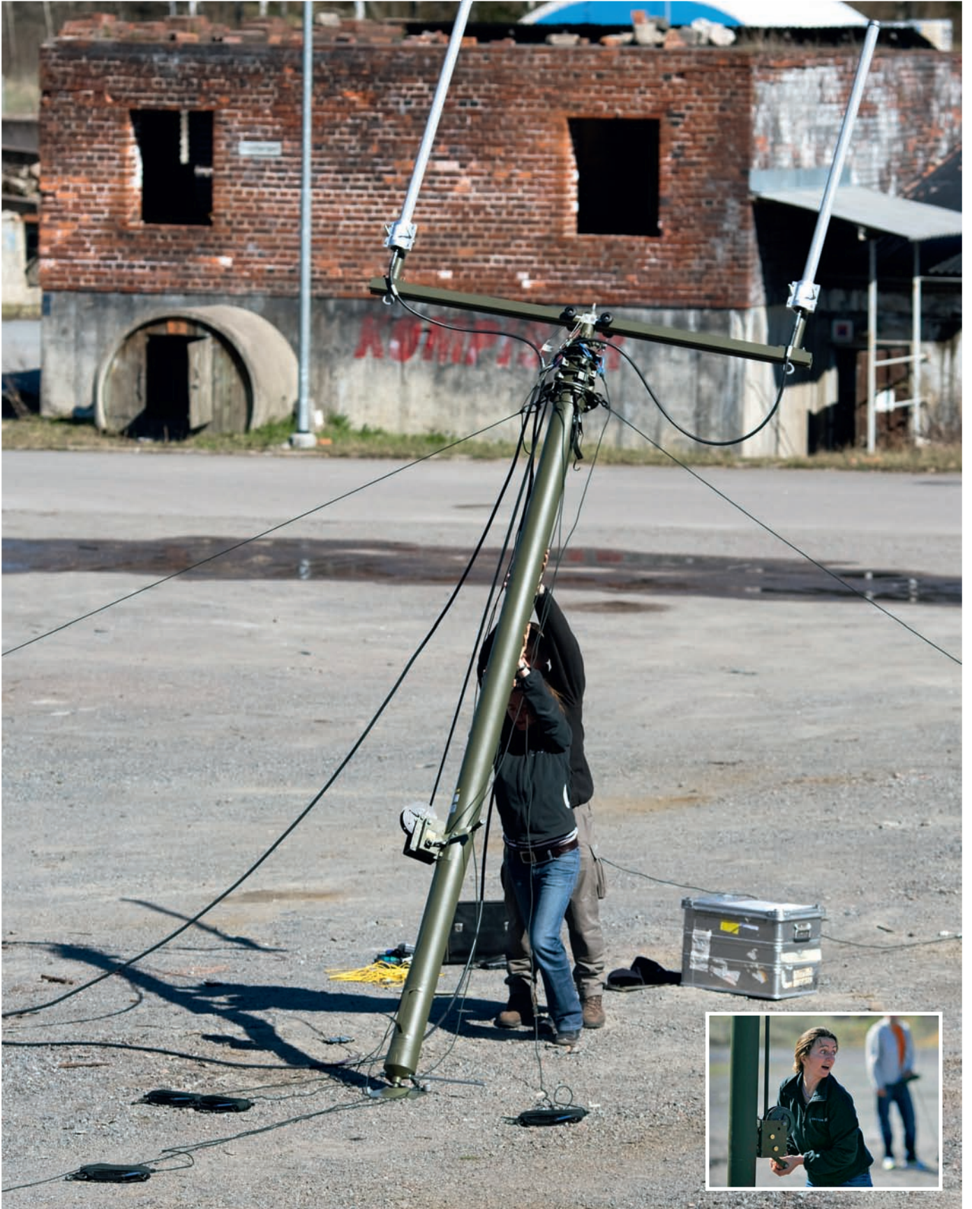
It takes just a few minutes for the rescue team to raise the mast for the QuicLINK system. Once the supporting cables are secure, Ester Gonzalez de Langarica from Ericsson Response winches up the antennas to a height of about 15m, which provides good coverage.
