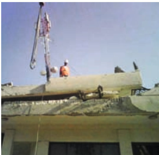
The radio base station and mast on the roof of a house in Port-au-Prince that was hit by the earthquake. The roof gave way but the site remained intact.
