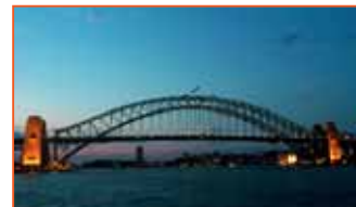
A photo of Sydney Harbor Bridge, taken during work recently.
