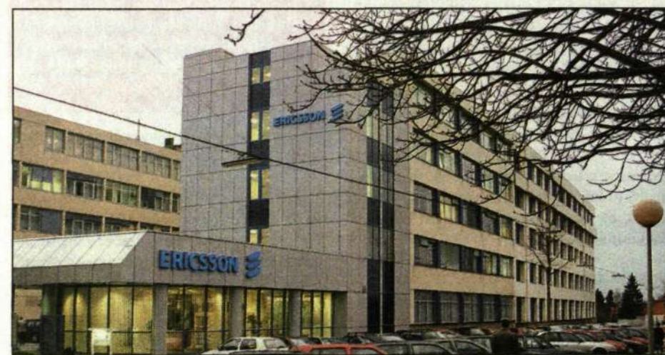
Ericsson Austria's new facade on Pottendorferstrasse in Vienna, where BusinessPhone is headquartered. The building was commissioned by Ericsson prior to World War I. Schrack took it over in the late 1930s. Ericsson Schrack was formed in 1994 when Ericsson acquired Schrack, and in 1996 the name was changed to Ericsson Austria. Photo: THORD ANDERSSON
