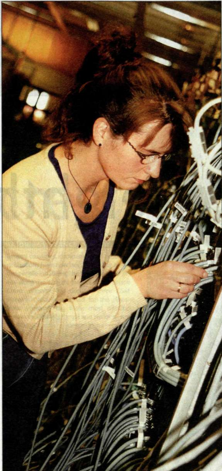
Camilla Lundstedt's job has become more interesting and rewarding since node assembly workers were given comprehensive workplace responsibility. As a node assembly employee, Camilla works with the equipment at all stages, including final installation.
