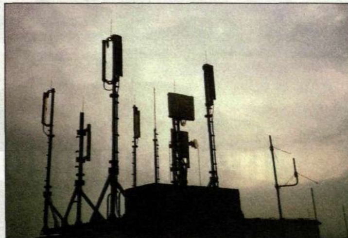
Ericsson's adaptive antenna technology (in the middle) improves both the capacity and speech quality of GSM networks. A test system is now in operation on a commercial network in Germany.
