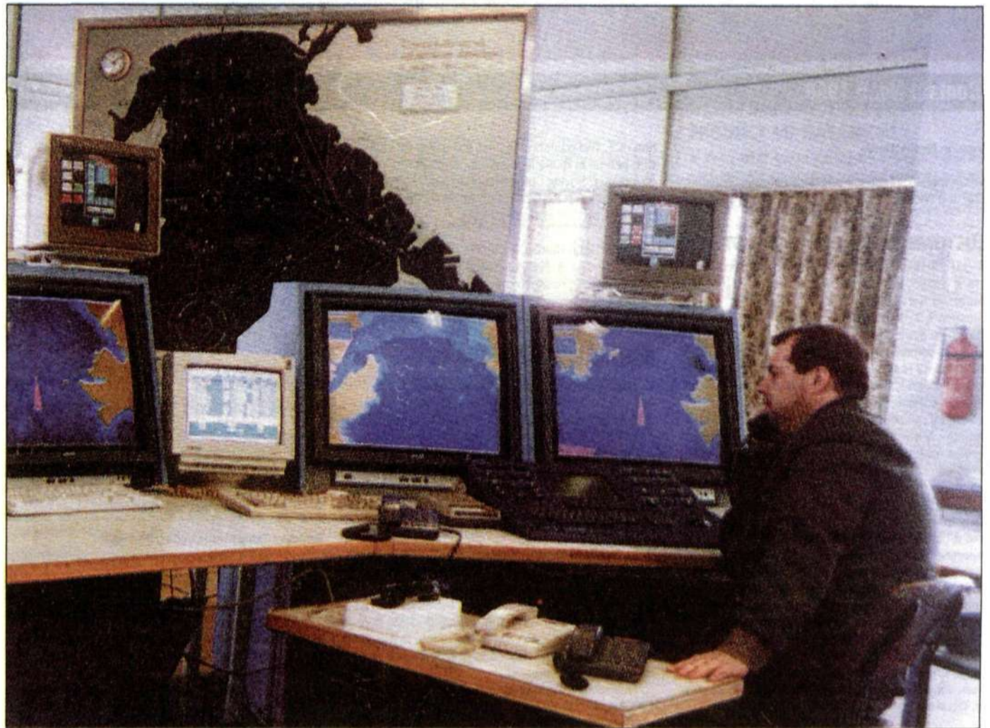
One of the operations sites used in the coastal radio system in Vladivostok, which features radar and telephony equipment from Ericsson.
