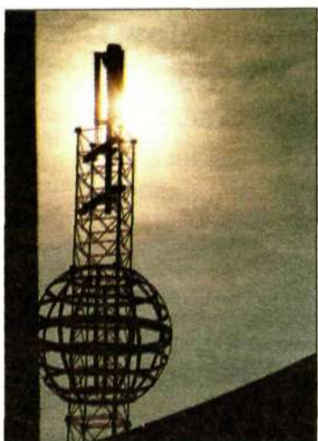
The antenna for the WCDMA base station towered between the two halls at CeBIT, where the Ericsson stands were located. Photo: Lars Åström
