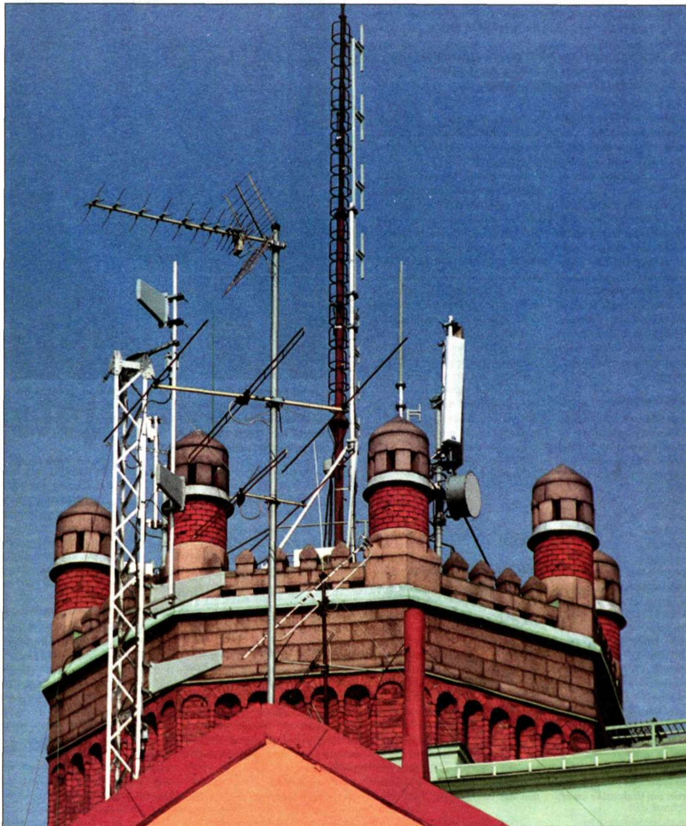
Equipment for mobile telephone networks is an established feature of the Stockholm skyline nowadays. A study carried out by Ericsson and AT&T shows, however, that the networks have limited environmental impact. Photo: Lars Åström
