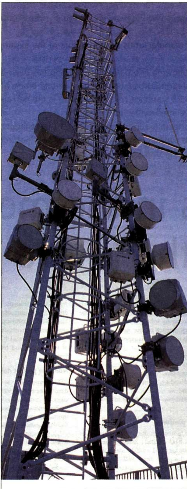
The revolutionary feature of MINI-LINK was that parts of it were located outdoors, adjacent to the antenna. In this way, a coaxial cable was able to communicate between the modem and the antenna.
