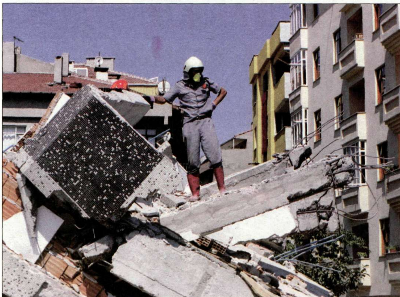
Tens of thousands of people died as a result of the earthquake in Turkey. Ericsson was present from day one to restore the mobile network which was damaged in the quake. Communication needs were immense, and Ericsson distributed mobile phones to rescue workers and the communications centers that were set up to enable victims to contact the outside world. Photo: Lars Åström
