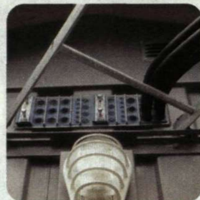
Rox System cable entry seals have become a popular standard within the telecom industry.
