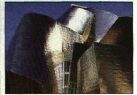
The undulating outer walls of the Guggenheim museum in Bilbao, Spain are covered in shiny titanium. The building's organic form is heightened through a combination of water reflections, glass and sand-colored stone. Photo: Erika Barahona
