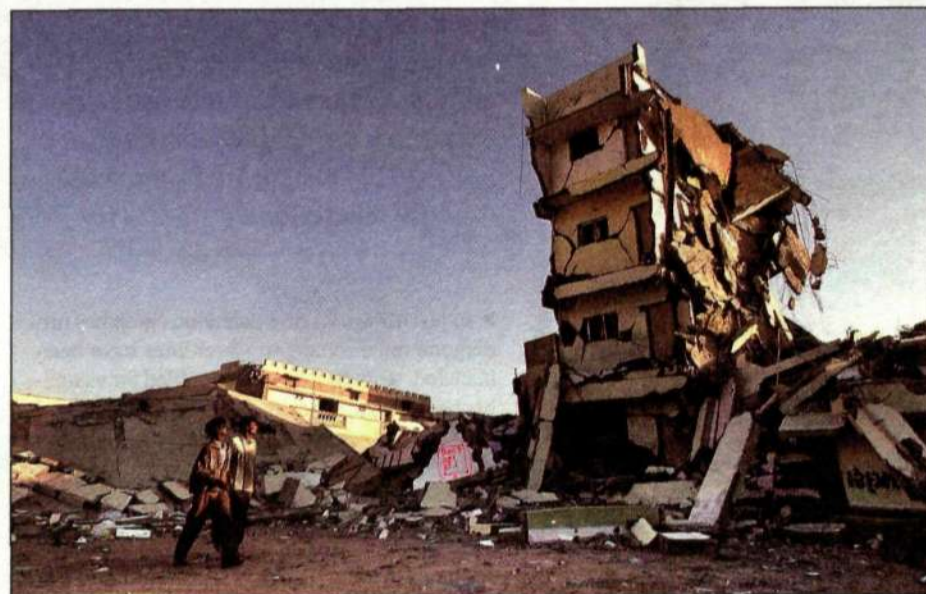
A couple of passersby look at a destroyed building where they used live in the town of Bhuj, in Gujarat state, which along with the entire northwestern India was hit by a massive earthquake 26 January. Photo: Pressens Bild/Arko Datta
