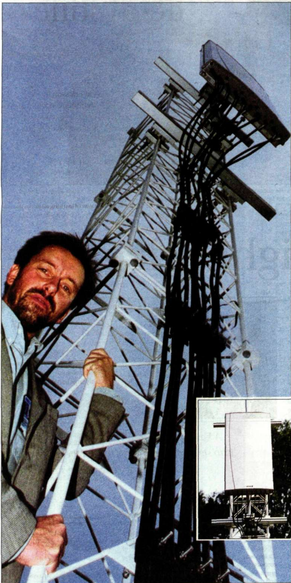
The secret lies in the wide antenna. "Using adaptive technology, such as dividing the cell into eight parts, we can reduce interference and more than double the capacity of a network," says Johnny Widén of Ericsson Microwave Systems. Photo: Niclas Henningsson
