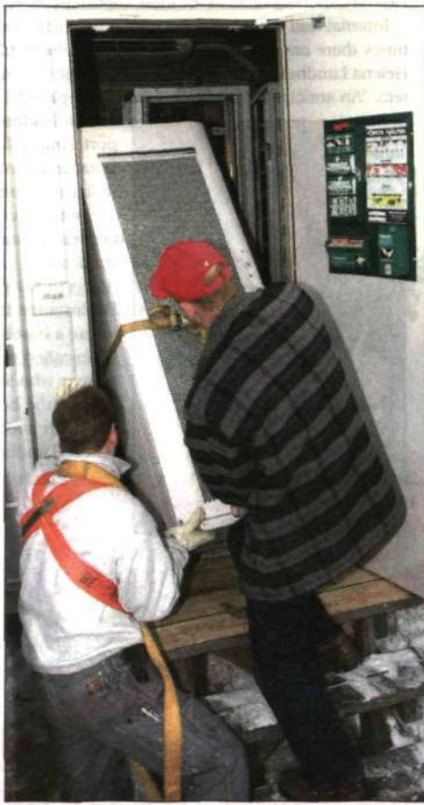
The Nordic region is well on its way in the 3G race. Yet another of the base stations that will serve the Swedish 3G network is installed on a roof in Stockholm.
