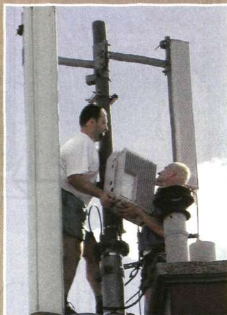
Mobilcom in Austria is the first operator in the world to install Ericsson's new RBS 3402 WCDMA base station in its network. The new base station makes it easier for a customer to quickly provide mobile coverage in, for example, an urban environment.
