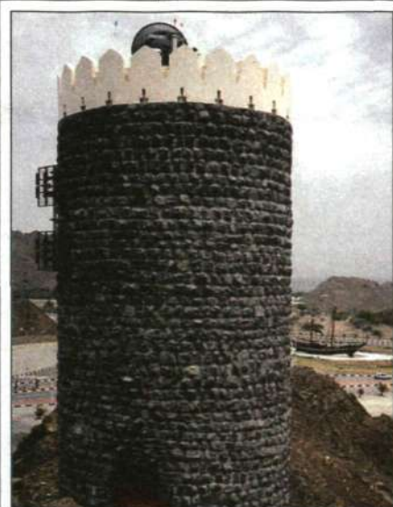
The rules in Oman state that base stations have to melt into the landscape. That explains this "antique" base station from 1988.
