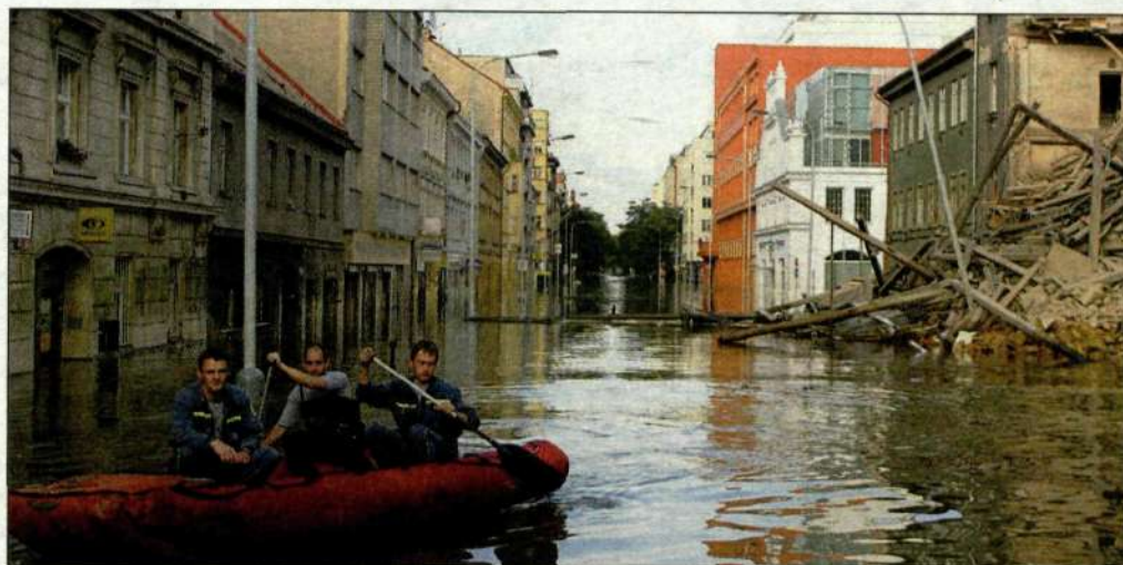
The Karlín district of Prague was one of the worst hit areas. Because the floodwaters have undermined buildings, the district has been cordoned off.
