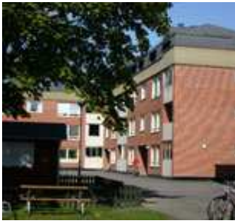
Figure 9. Field trial building, Hudiksvall, Sweden
