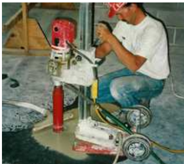
Figure 1. Core drilling
