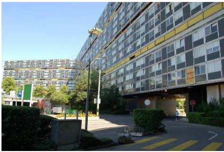
Figure 10. Field trial building
