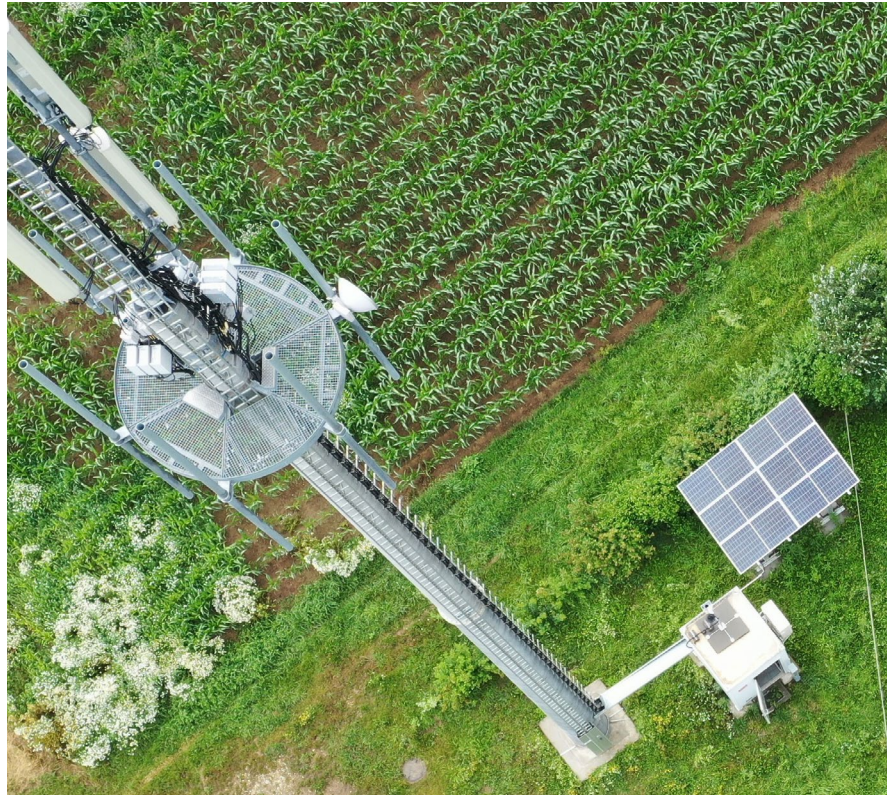
Ericsson and Deutsche Telekom have partnered to bring solar panels to a RAN network site. Image source: DFMG Deutsche Funkturm GmbH
