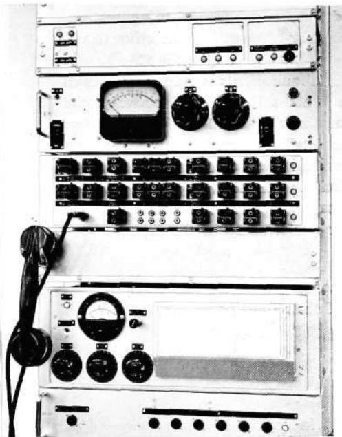
Fig. 6 v.u. meter, U-link panel and current distribution panel
