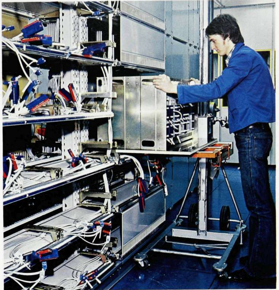
Fig. 7 Equipping a row section. The central processor is slid into position
