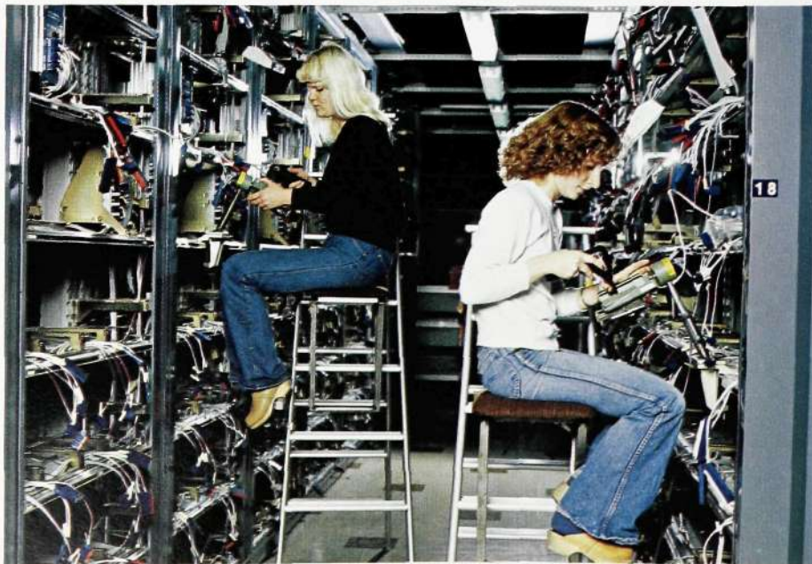
Fig. 6 External cables are connected to plugs by means of wire wrapping
