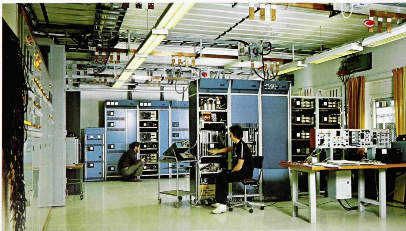
Fig. 1 System test room. The panels to the left are used for AC distribution. The bars for high direct currents are run across the ceiling. A small selection of the power supply equipment developed and manufactured by LM Ericsson can be seen in the background
