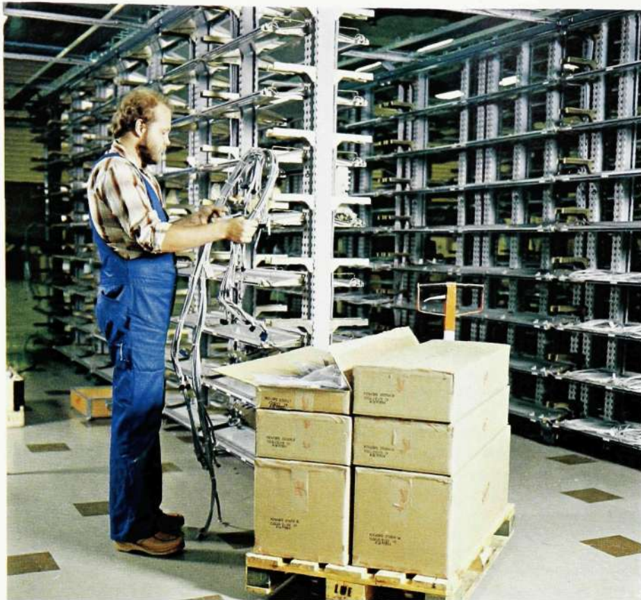
Fig. 4 Installation of cable trunks straight from the package. The trunks are packed and marked in the order they are to be placed in the cable section, which eliminates much handling and identification work
