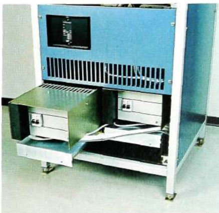
Fig. 9 Two transformer units, with the front plates removed, seen from the front in the rack. All 220 V connections are efficiently encapsulated and protected from accidental contact. The units are FI marked (class 2 insulation)
