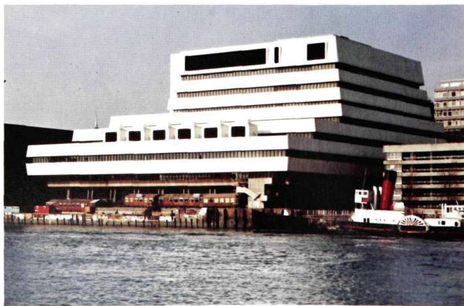
Fig. 1 London/Thames International Switching Centre (ISC) is situated on the north bank of the River Thames
