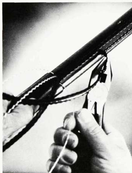
Fig. 2. Stripping the outer sheath and exposing the screening wires
