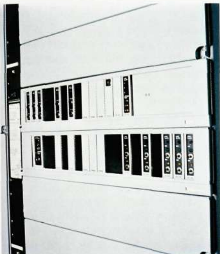
Fig. 12 Partially equipped protection switching equipment in a repeater station
