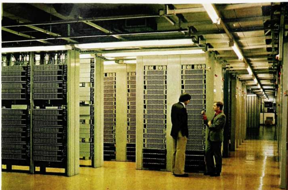
Fig. 10 AKE 132 with CCITT6 in the London/Thames ISC will provide high quality international telephone service
