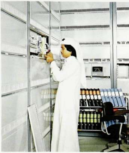
Fig. 4 Inspection of a magazine in the transit exchange in Riyadh
