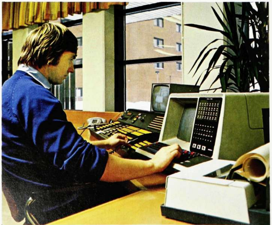
Fig. 1 Operator's position. A control panel gives a survey of the alarm situation. The visual display screen shows the recommended action as regards incoming alarms. All measures are recorded on the printer
