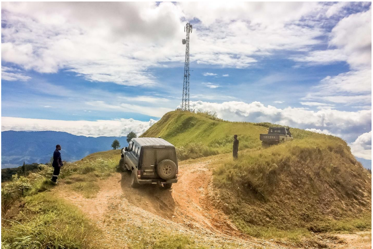
Figure 1. Ericsson's Authorized Service Provider Employees, accessing to network site in Papua New Guinea for maintenance.
