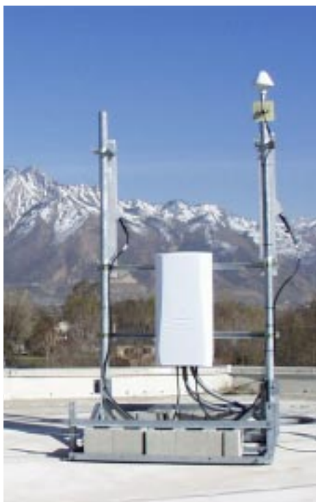
Figure 4 The Ericsson RBS 1106—typical installation configuration.
