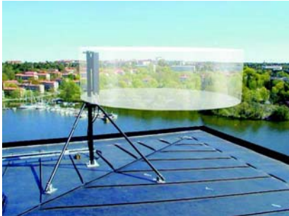
Figure 7 RF exposure compliance boundary for an antenna connected to an Ericsson RBS 3202 (UMTS) base station.
